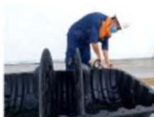
5. Sealing tape on the edge of the bottom cover (No need to tear the upper layer)
