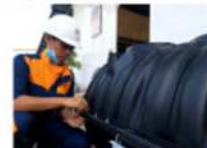
8. Sealed by bolts & nuts
