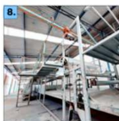
Roofing/Cladding Quantity : 1 Machine
